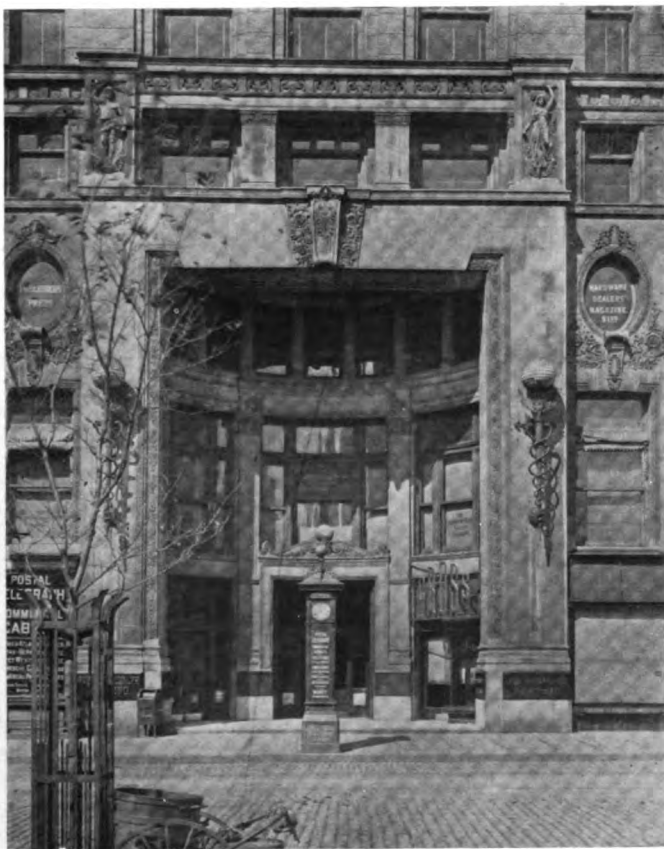
Postal Telegraph Building—Main Entrance.
